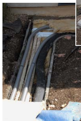
Concrete ducting enclosing a range of pipes. Note insulation placed above and below the pipes. Inset, with the lids added, later to be covered with gravel.
